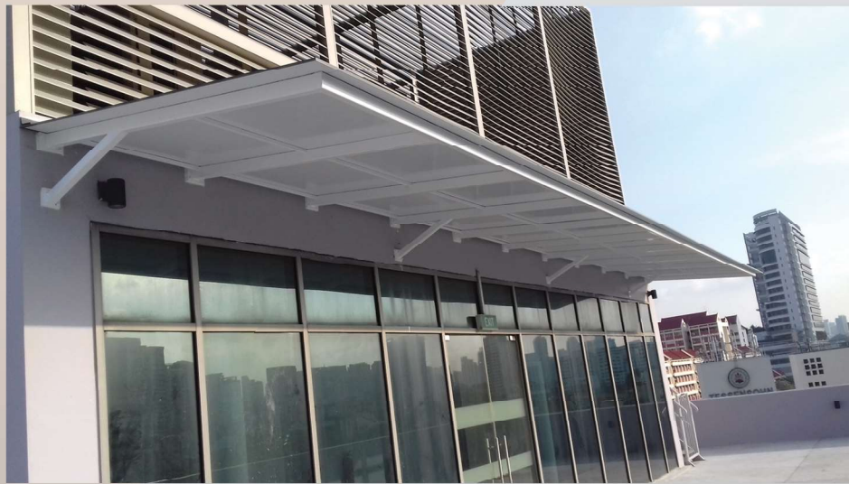
Aluminium Composite Panel (ACP) Roofing
