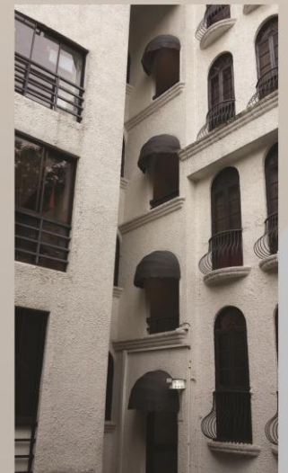
Customised Steel Canopy
