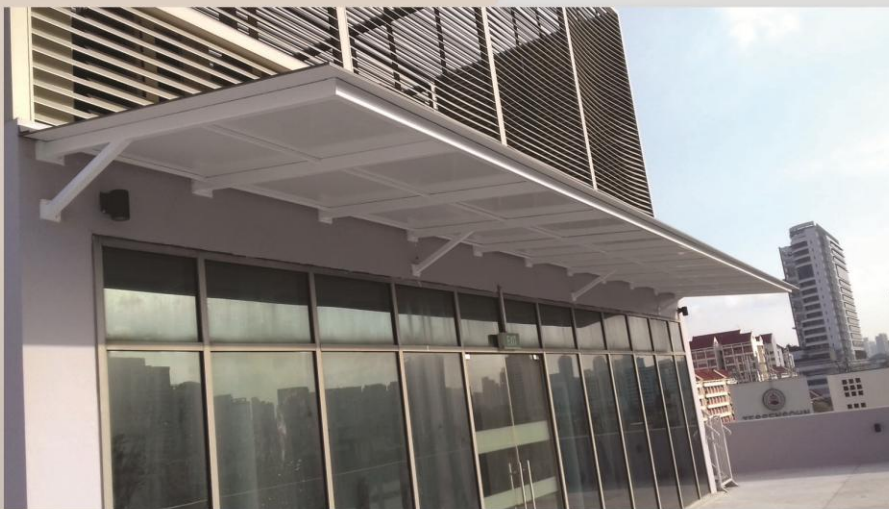
Aluminium Composite Panel (ACP) Roofing
